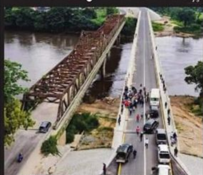
Newly-constructed double Lane Bridge at Ekot-Mfum, Nigeria
